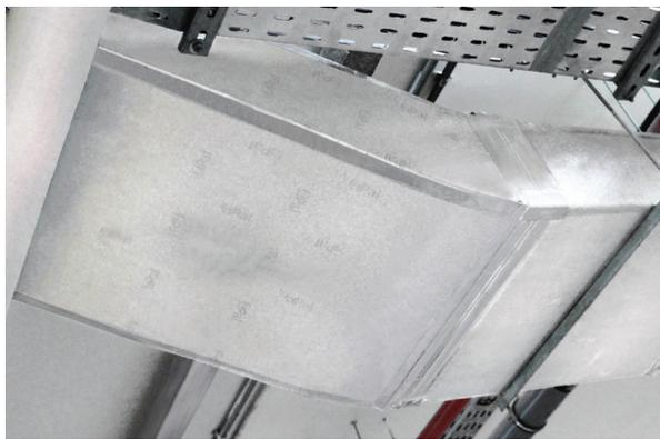
Kingspan PalDuct systems have been the pioneer in pre-insulated ducting. Pal was the first company in the world to introduce the innovative and revolutionary rigid pre-insulated ductwork as an alternative to sheet metal ductwork. It was invented by Claudio Ferraro of Bologna, Italy in 1965.
